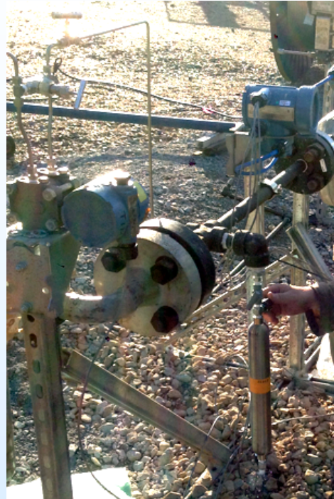
Gas collection into steel canister directly at well fitting.
