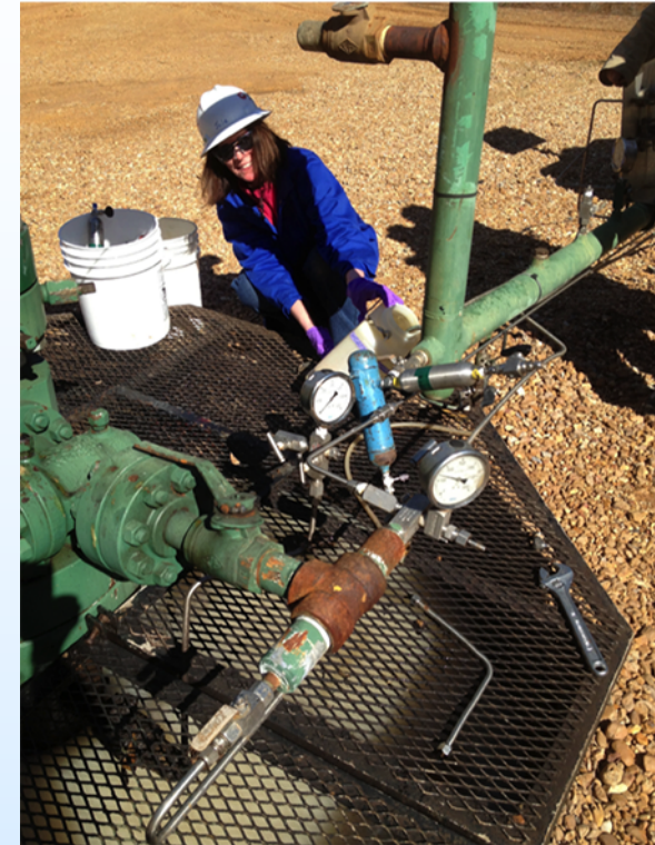
Gas/water separator for gas collection. Fluids were collected into a carboy.
